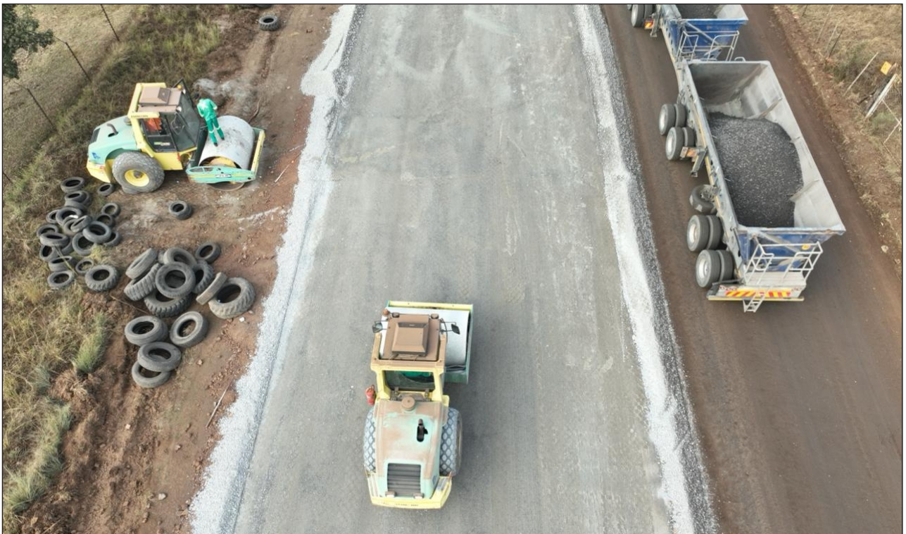
The 26-kilometer segment from Road P51 to the P2/4 (R104) connecting Majakaneng and Berseba in Madibeng Local Municipality has reached a 41% completion milestone. These efforts involve applying an asphalt overlay to specific areas and undertaking patch and reseal work on the rest of the road. MEC Sempe Elizabeth Mokuu's oversight visit on this road project in the Bojanala District was aimed at monitoring progress.
