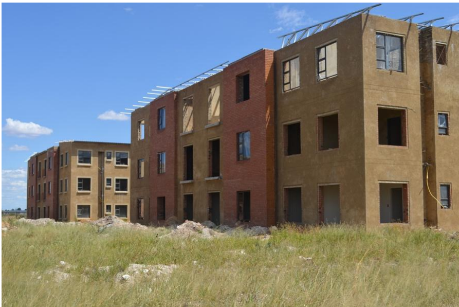
The incomplete structures of social units.
