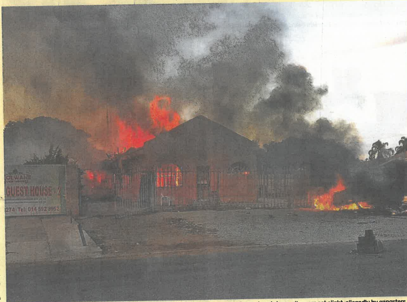
CRIMINAL ACTIVITY: Eight buildings, including residential houses and guest houses in Rustenburg's inner city, were set alight, allegedly by gangsters.
